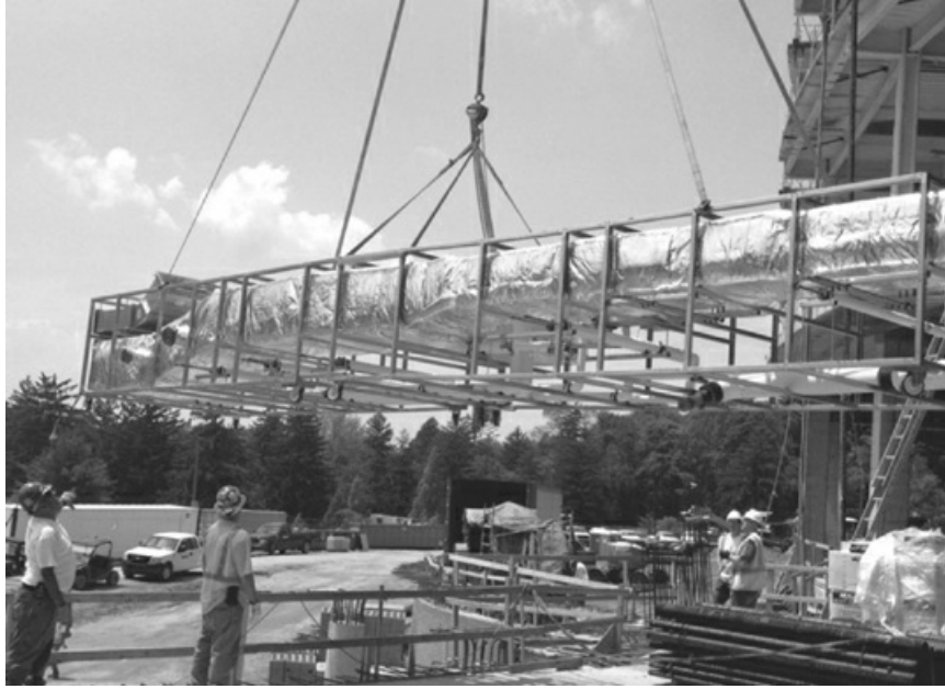
Figure 5.4 Installing prefabricated mechanical racks
